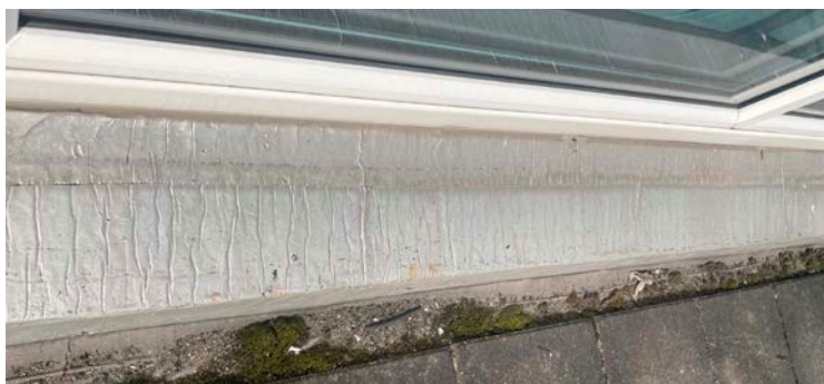
Examples of Sylglas™ Flashing Tape applications from the early 1990's, still in service. (photographed in 2024)
